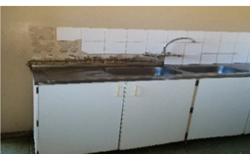
Broken tap, blocked drain and tiles peeling from the wall in the OT department
